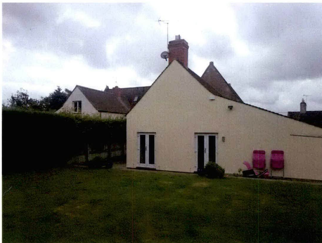
Existing photograph of rear from rear garden of no 1 The School showing large extension
